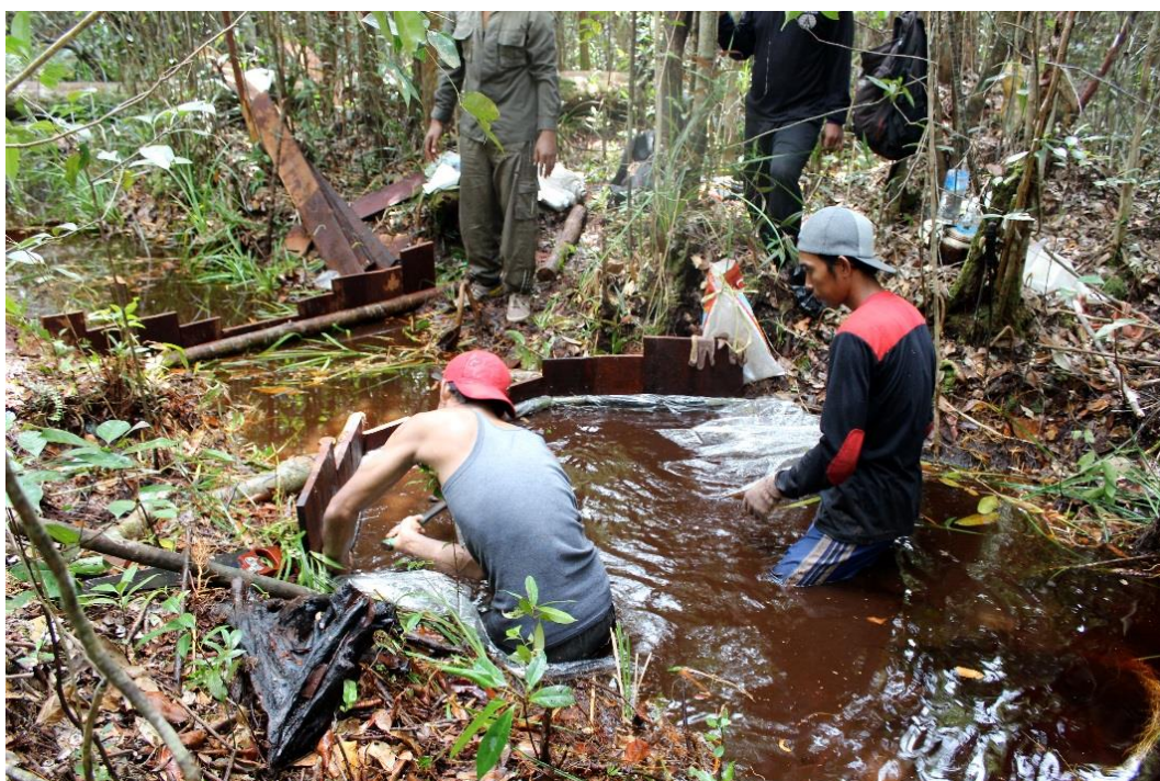
Figure 32: Building a dam in a drainage canal in Sebangau peat-swamp forest in Indonesia. Photo by BNF.
