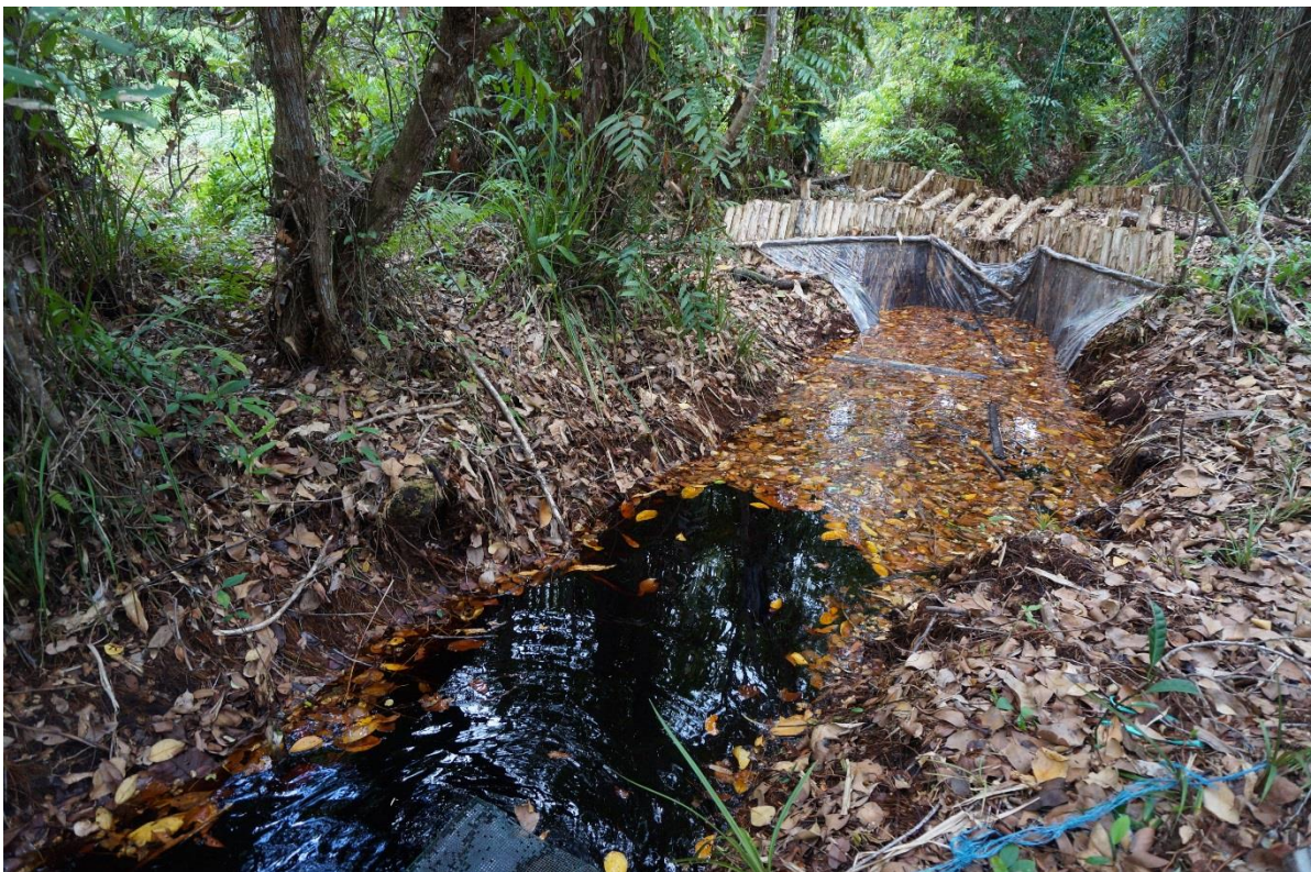
Figure 31: A dam blocking a drainage canal in a tropical peat-swamp forest in Indonesia. Photograph by Sara Thornton.
